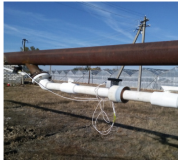
Fig. 6. Exterior of tube supplying geothermal water and device with electronic components installed on it
